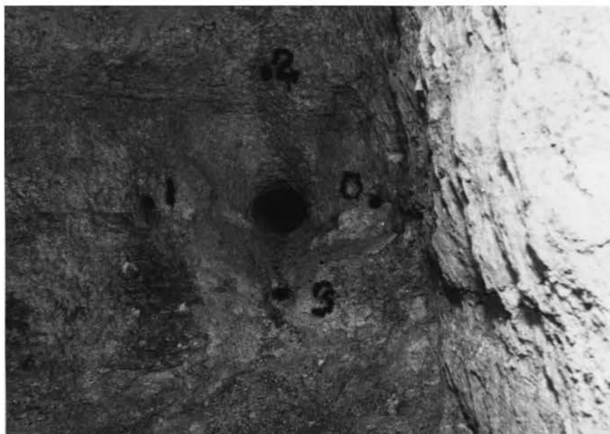
Photograph 14A. Pattern of Cut Holes For Round Number 14.
