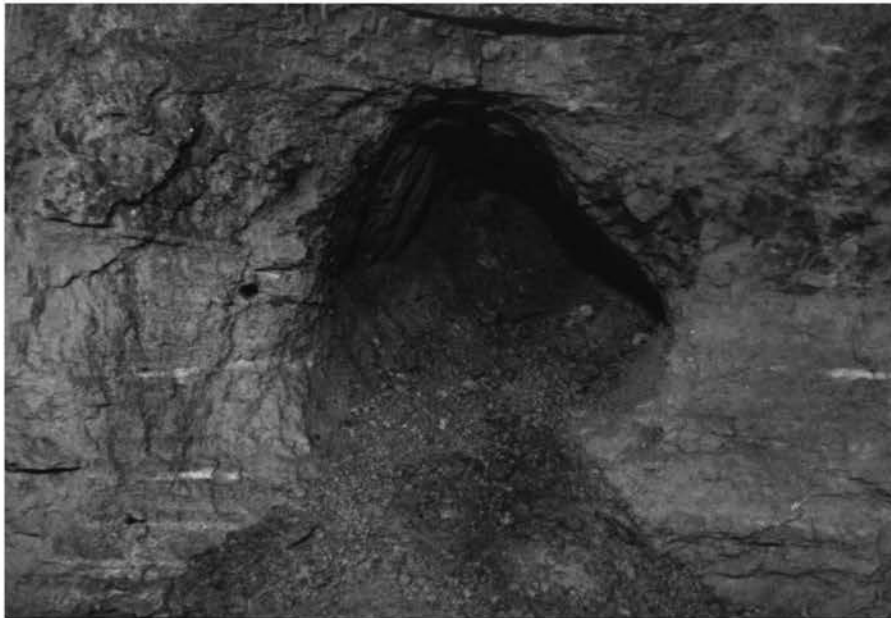
Photograph 4. Results of Burn Cut Number 4
