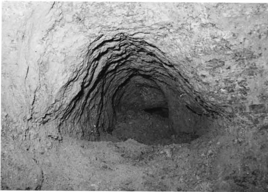
Photograph 11. Results of Burn Cut Number 11. The Bottom of the Cut Visible in the Picture is 12'4" From the Original Face of the Drift.
