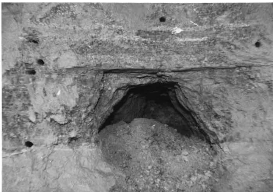
Photograph 7. Results of Burn Cut Number 7 Bottom of Cut is 9'9" From Original Face of Drift
