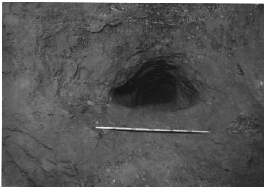
Photograph 15. Results of Burn Cut Number 15. Visible Depth of Cut is 14 Feet.
